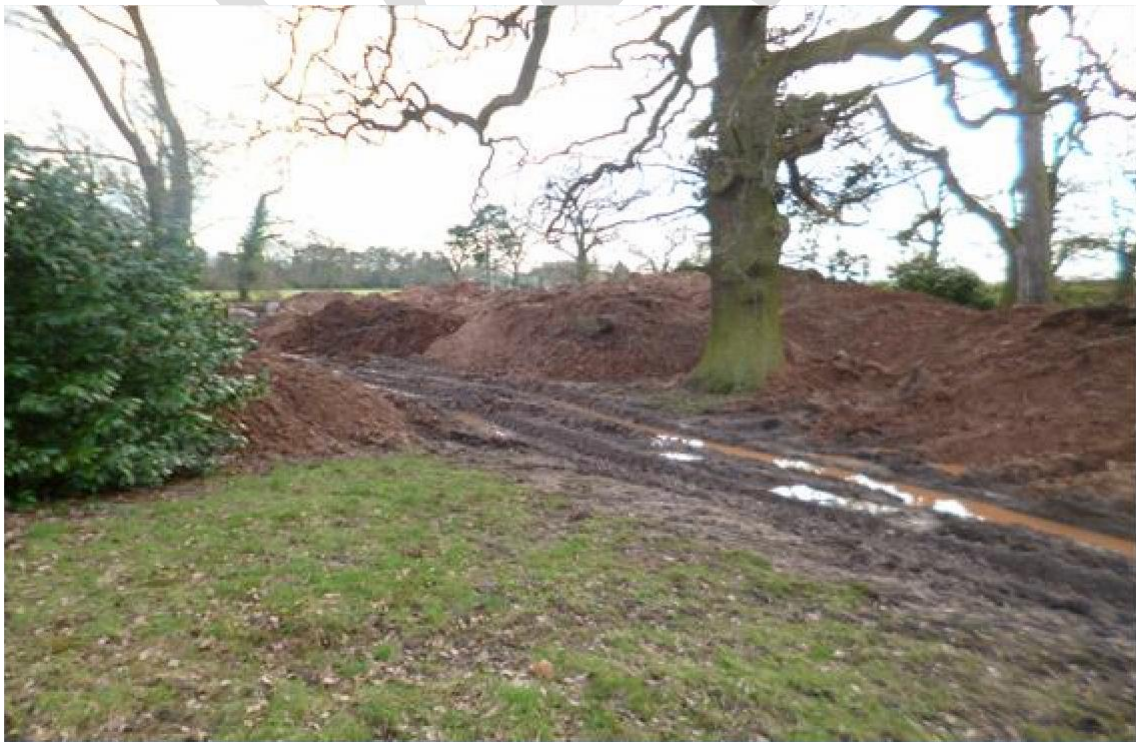
Damaged soil structure from the passing site vehicles within the Root Protection Zone.
